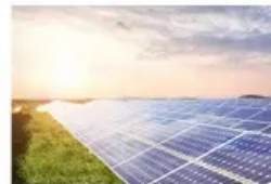
Energy Storage System
