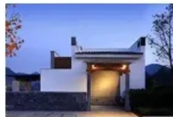
Household Energy Storage
